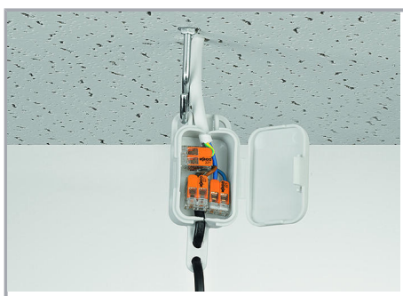
Pendant light connection in a suspended ceiling
