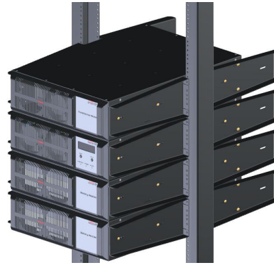
FIGURE. 6: INSTALL REMAINING T1000 MODULES
