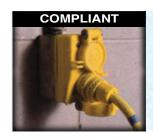
3) Do we have 15 or 20 amp, 125 or 250 volt receptacles installed in wet locations that are NOT weatherproof with or without the attachment plug inserted?
