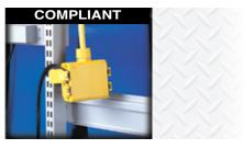
4) Are pendant applications (flexible cord drop from the ceiling without structural support) using boxes that are NOT listed for pendant applications?
