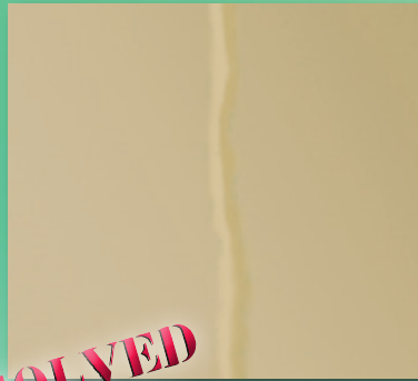
Tunneling or buckling
