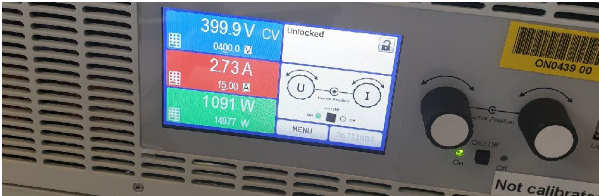
Figure 23. DC Power Supply Reading @ 1 kW.
