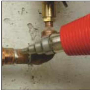
Solder Copper Pipe
