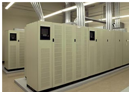
Uninterrupted Power Supplies
