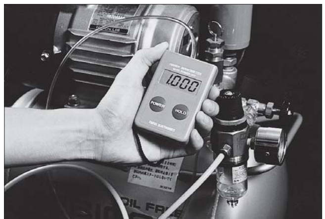
▲ Measurement of source pressure from a compressor.
