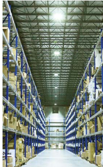
MedSafe Warehouse Facility
