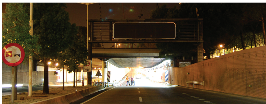
T-Max fixtures by Carandini using LUXEON M LEDs were installed in el Túnel de la Vila Olímpica. Carandini provided a customized design, which minimizes the stark contrast between outside daylight and the dark tunnel.
